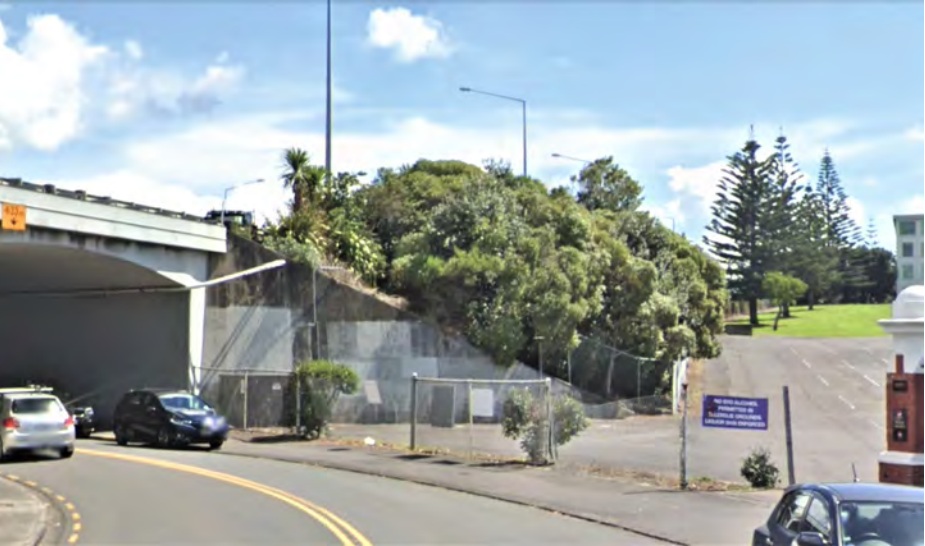
MITCHELSON STREET UNDERPASS LOOKING ALONG SW BOUNDARY
