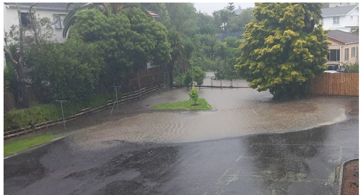
Pipe upgrades increase drainage capacity that improve safety on roads and around buildings in medium sized 1 in 10yr storms.
