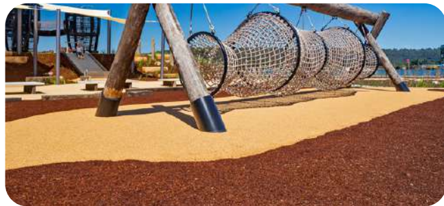
Playground surfacing - wetpour
