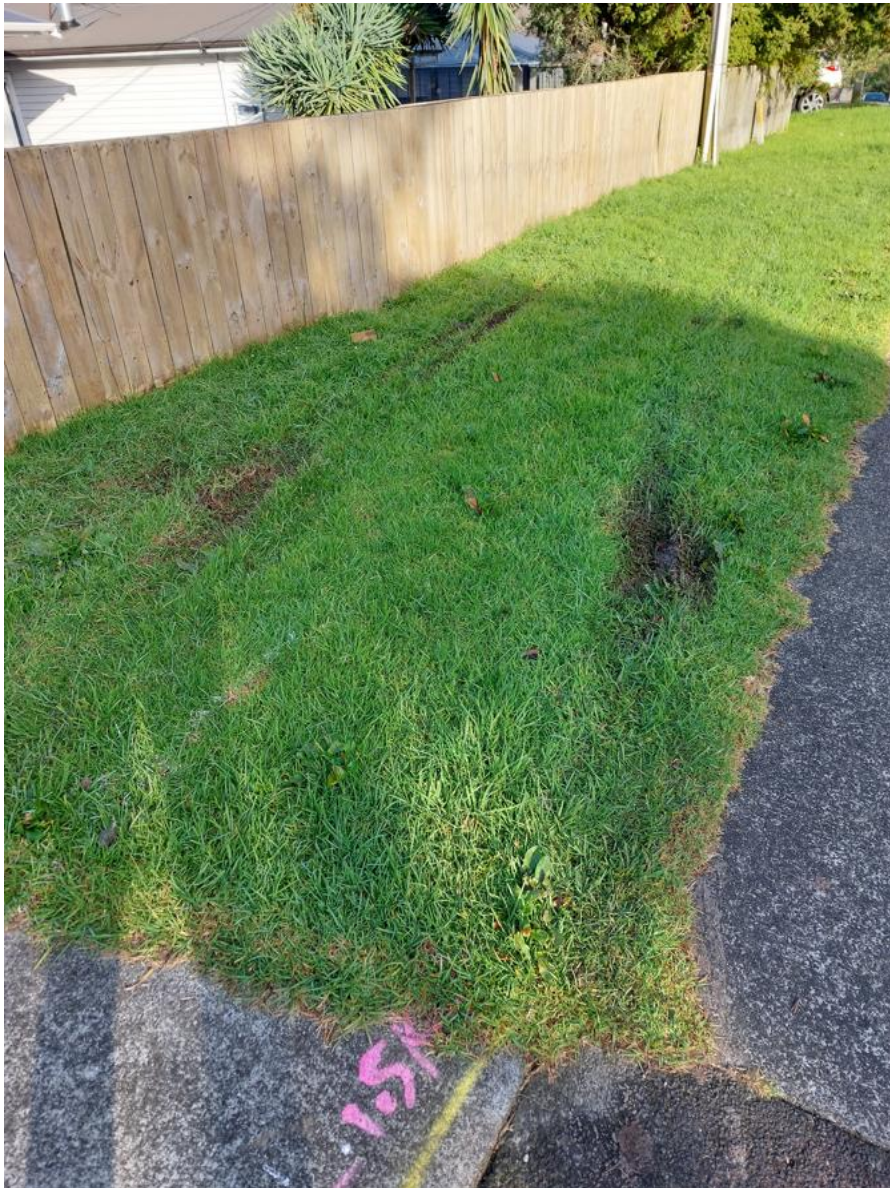
Image 7.5 – Damaged road berms.
