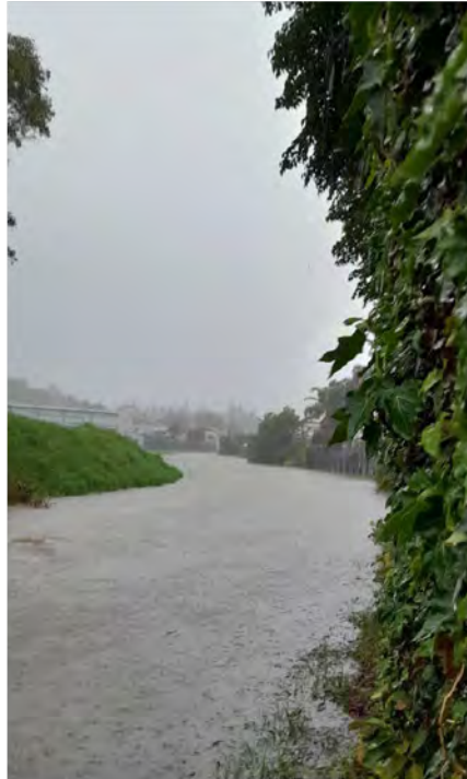
Photo 2. Back Culvert, Glendowie College - 9 th May 2023
