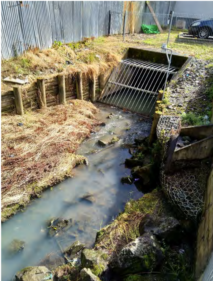
Fig. 1 Culvert at car park is currently cleared as of August 2023
