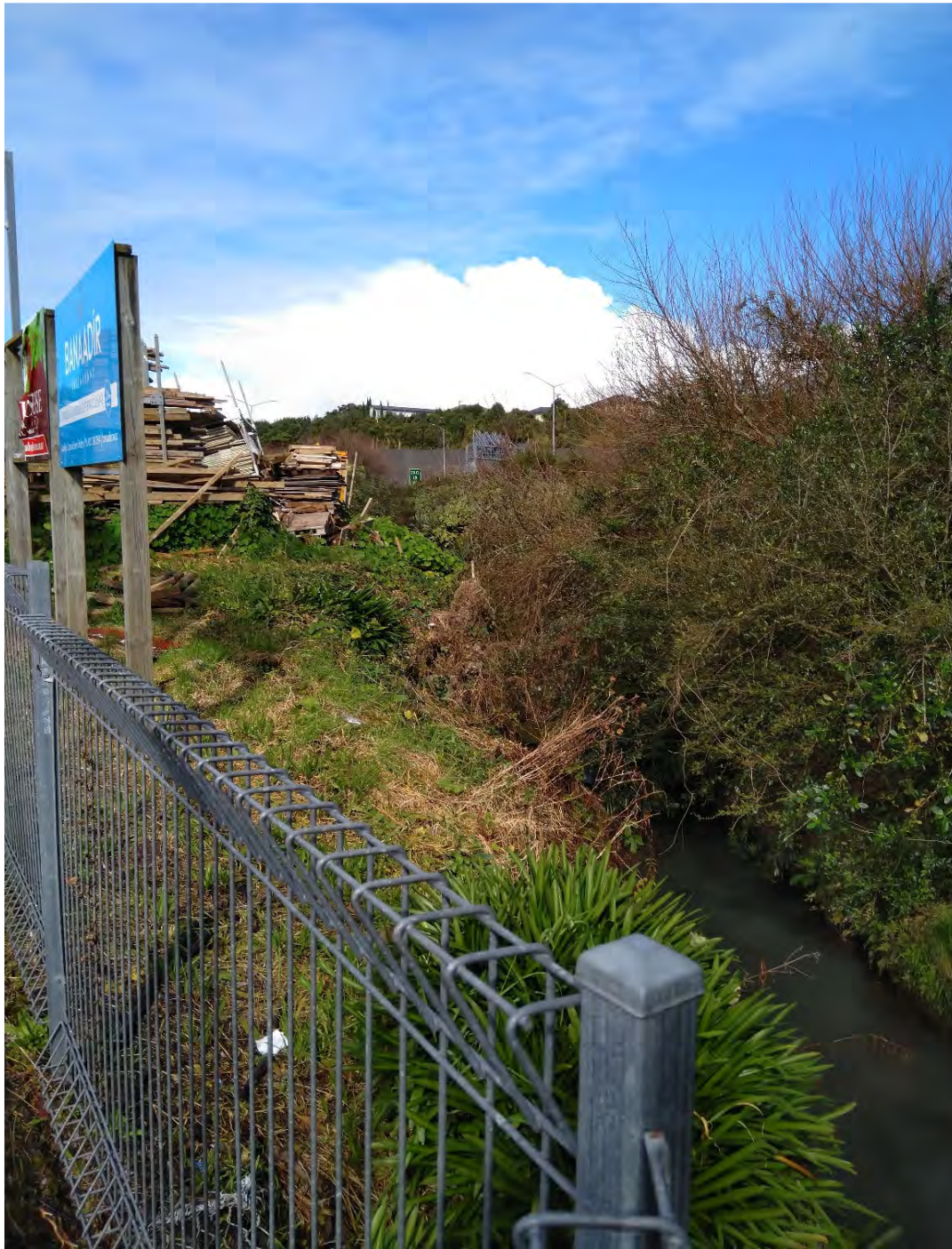
Fig. 4 Tributary behind Tulja Centre carpark, overgrown by noxious vegetation blocking the stream, mature vegetation indicates decades of neglect by AC, river margin is used for non-permitted storage, location is approx. 100m from culvert in Fig. 7
