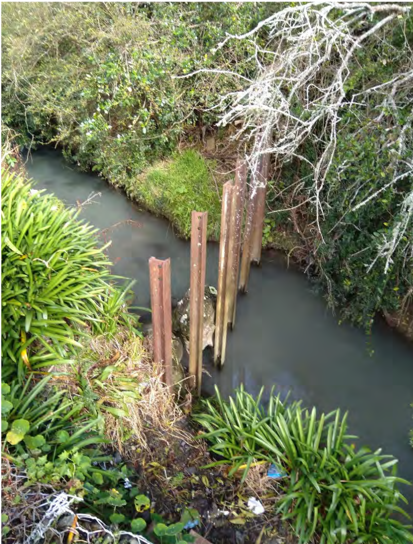
Fig. 2 Tributary adjacent to Tulja Centre carpark, location approx. 50m from culvert in Fig. 1
