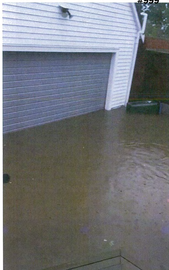
Flooding outside garage 27 January 2023
