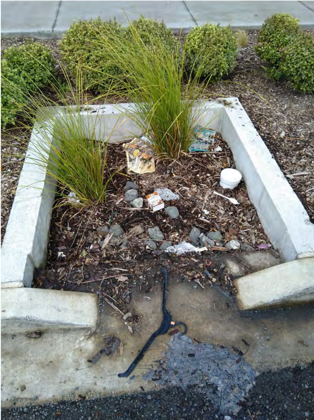
Fig. 5 recently installed stormwater drain inlet in Range View Rd/Owairaka, rubbish and construction debris block proper functioning,
