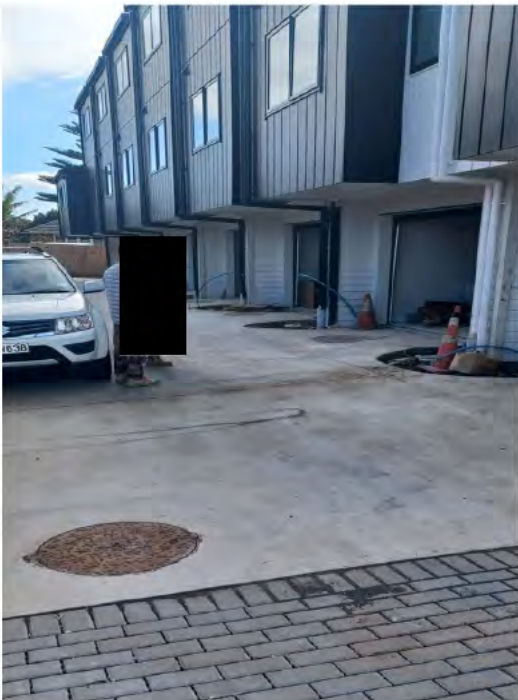
Where are the trees, the grass and the permeable surfaces. Perfect example of intensification causing issues.
