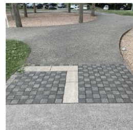
Existing site Pavers to be refurbished
