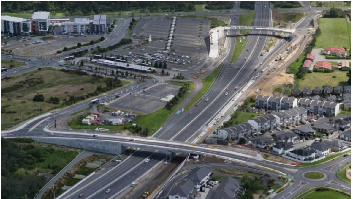
Figure 21 - October 2021 Waka Kotahi photograph 38 of progress at the Albany Busway Station and associated walkways and cycleway progress linking to eastern side Oteha Valley Road
