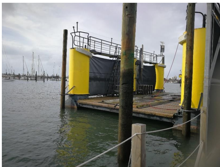
Figure 16: Floating Dock Services, Westhaven, Auckland.
