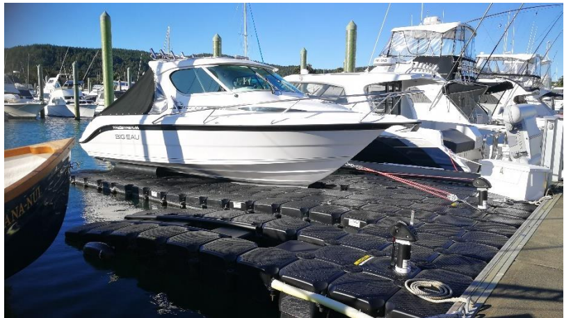
Figure 17: Dry berth, Whangamata Marina.
