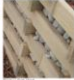
Timber Grid Wall
