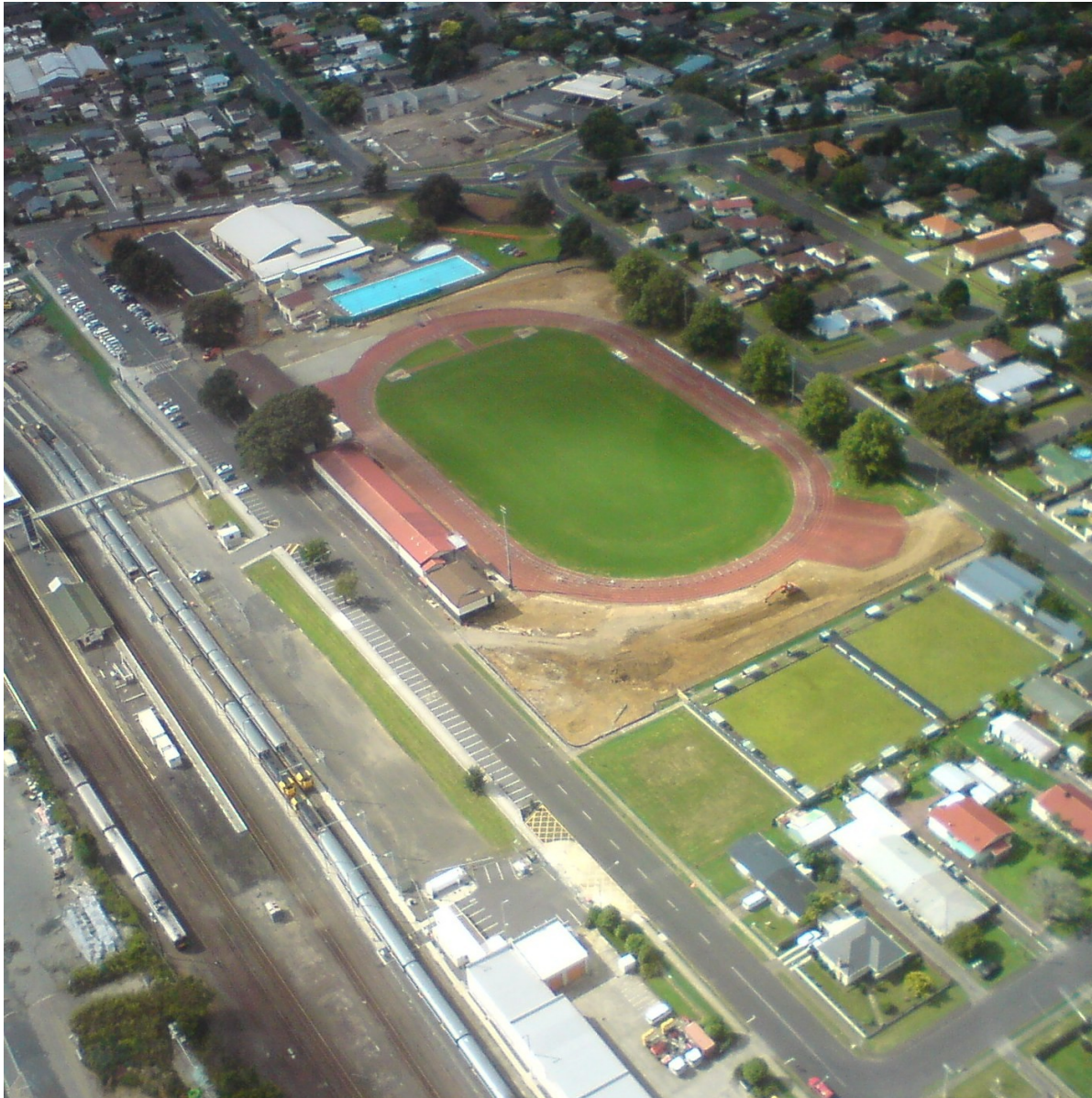
Massey Park during redevelopment in February 2011 - James Burgess
