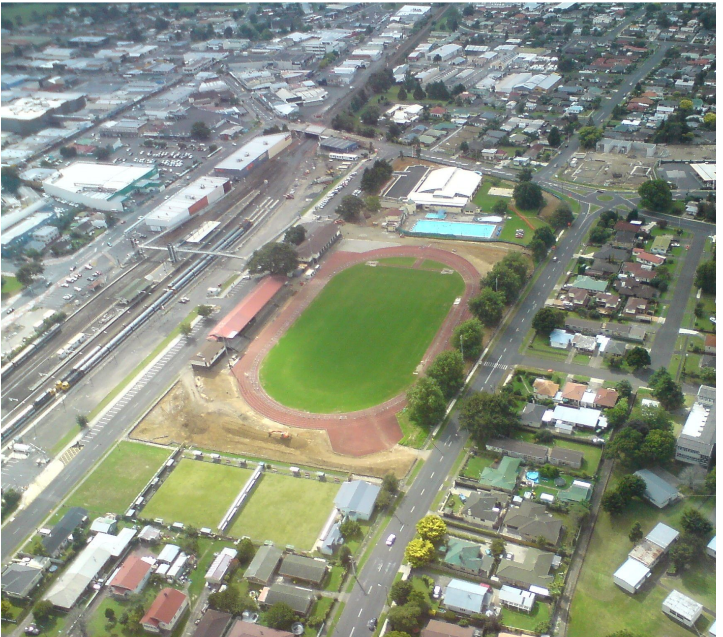
Massey Park renovations February 2011 – James Burgess
