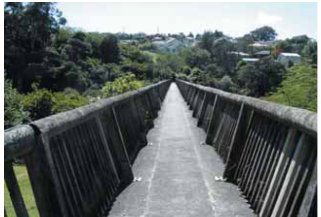
Connecting Bridge, Realm Esplanade and West Harbour Esplanade
