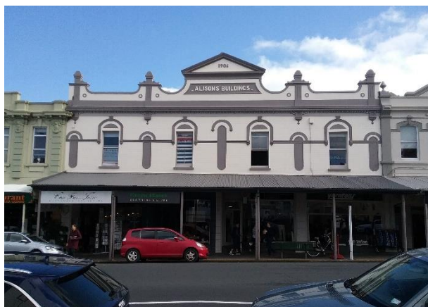
Figure 3: Alisons' Buildings, 73-79 Victoria Road
