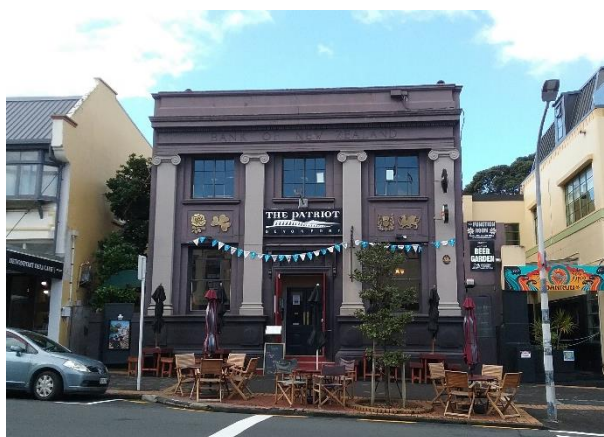
Figure 2: Bank of New Zealand (former), 14 Victoria Road
