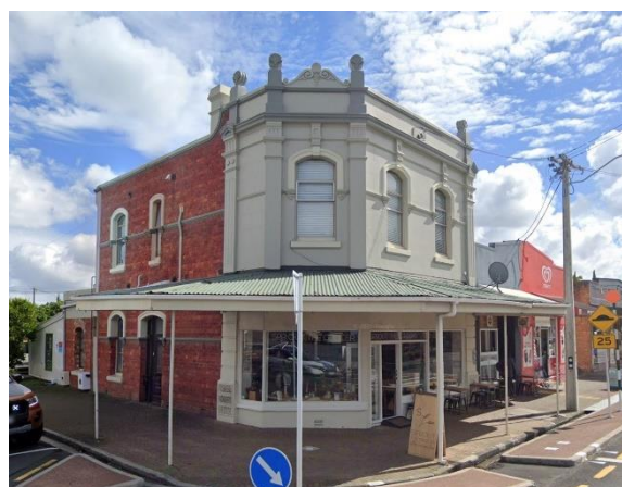
Figure 2: 100 Hinemoa Street, (Google Street View, April 2021)
