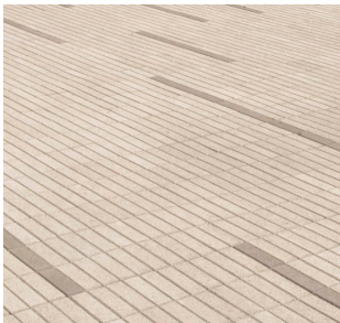
Raised table paving linking Sentinel Plaza
