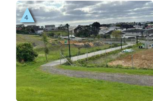
View of the AT path from the reserve
