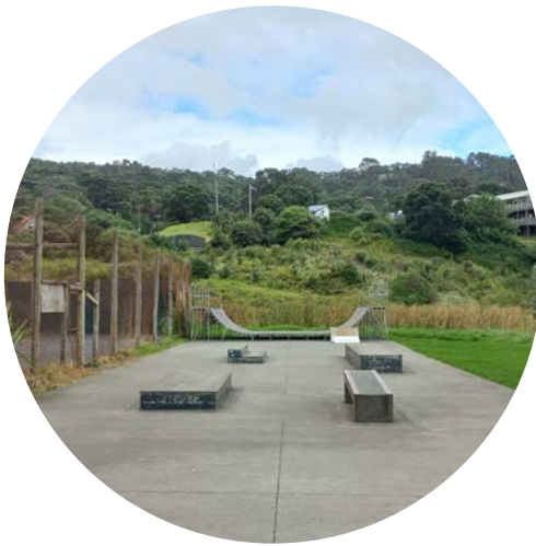
Rusted half pipe and lack of skate features
