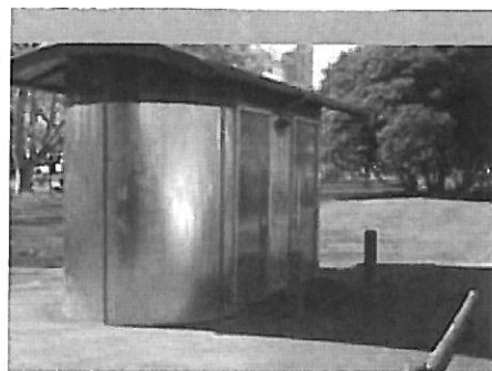
Toilets fronting Victoria Street West.
