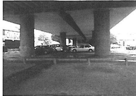
Parking beneath the viaduct overpass. Campbell Free kindergarten to the left.
