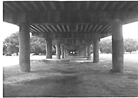
View under Southern Motorway viaduct.
