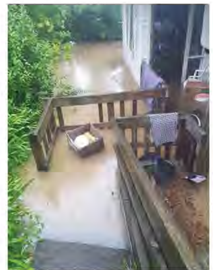
A flooded Visionwest property
