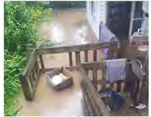
A flooded Visionwest property.
