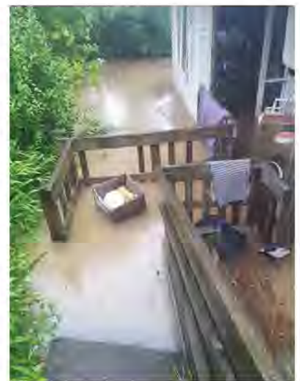
A flooded Visionwest property
