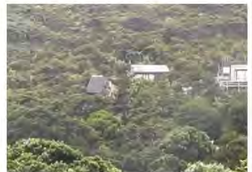
Landslip affected houses in West Auckland
