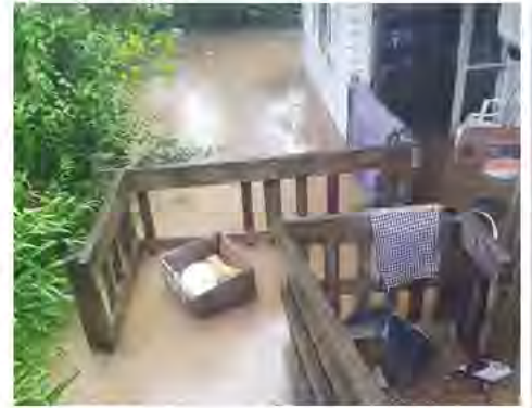
A flooded Visionwest property.
