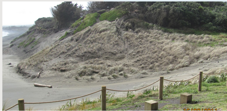
Right (top): Muriwai 2005 erosion of southern carpark area (pre managed realignment) source: Auckland council Right (bottom) Muriwai 2011, following dune restoration. Source: Auckland Council
