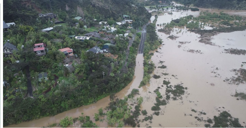
Left: coastal inundation Auckland's northern motorway, 2011
