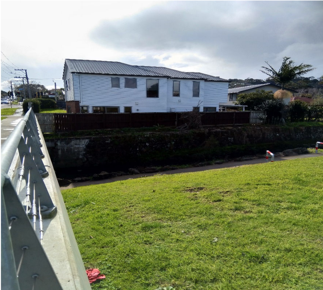
Fig. 8 South facing view of Example 2, in front are Te Auaunga/Oakley Creek, embankment wall with public walkway where recent flooding occurred, image is for the purpose of consultation only
