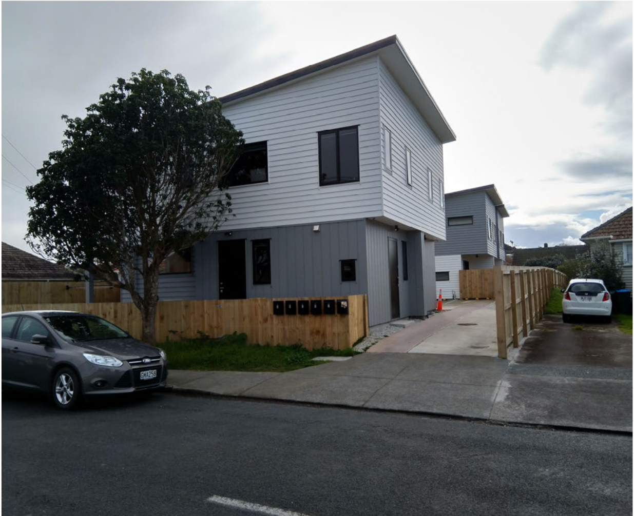
Fig. 10 Example 4 of impervious section exceeding AUPOIP requirements, 15 a-f Parkinson Ave in Wesley in the vicinity of Underwood Park, image is for the purpose of consultation only
