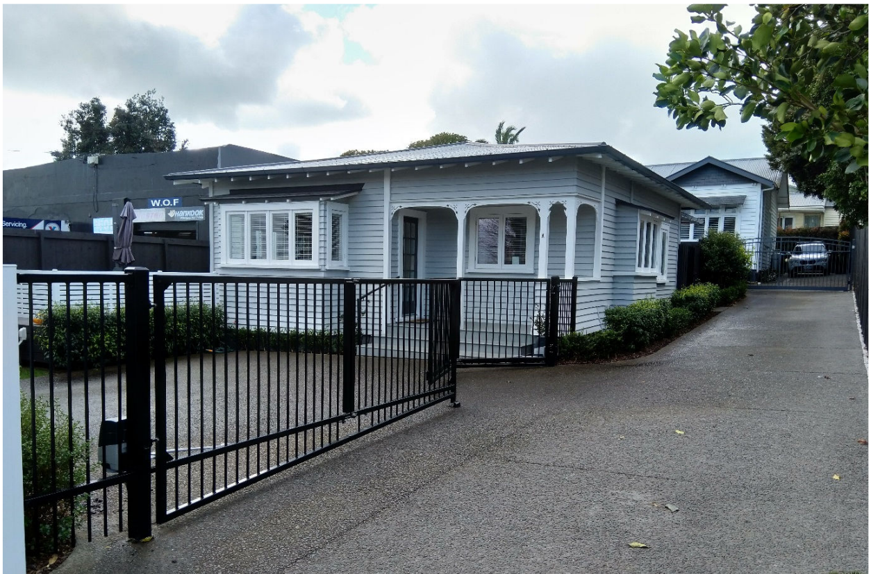
Fig. 6 Impervious surface in excess of est. 80% of property size due to subdivision, image is for the purpose of consultation under s82 LGA only, location in Owairaka,
