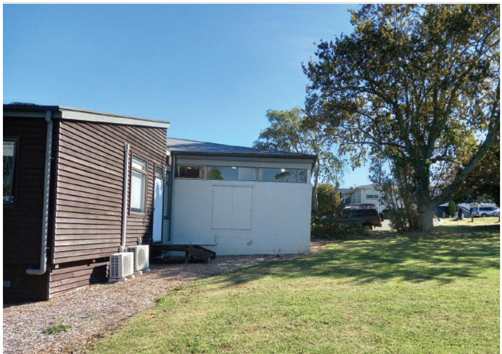
Lack of boundary treatment between St John's and park
