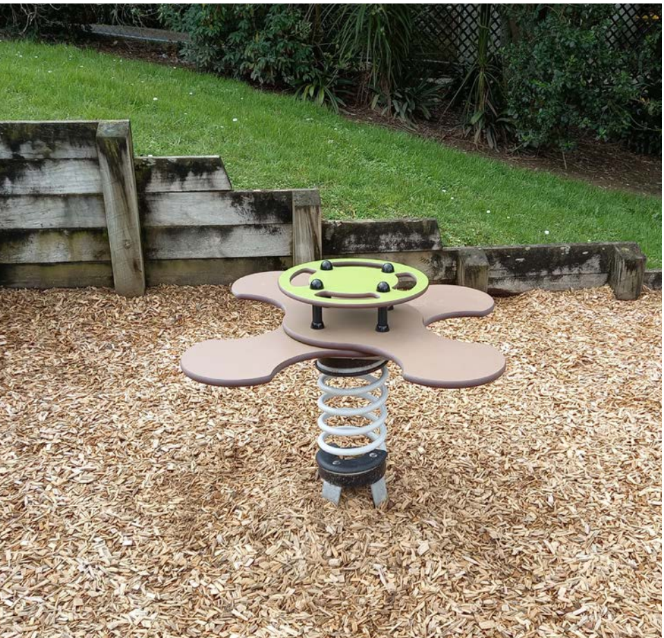
The springer is in good condition and can be retained
