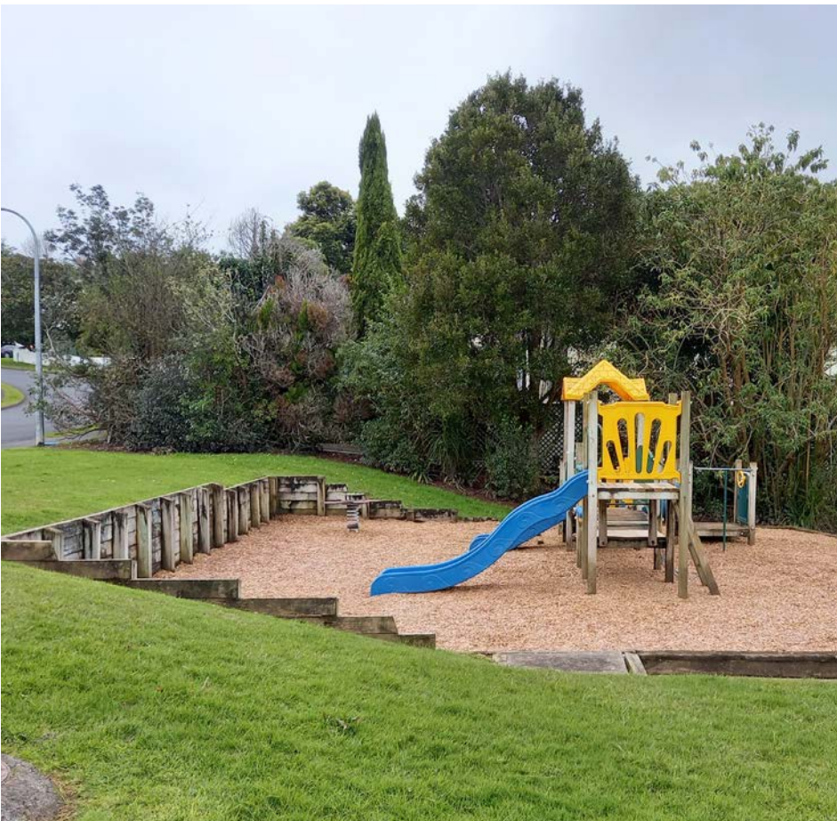
Existing timber retaining wall and raised edges
